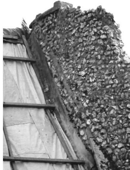
Pl.5 The east face of the ruined tower. The present roof apex can be seen to meet the tower south of the centre of the belfry cill. An earlier roof suggested by a line of remnant mortar weathering would have met it nearer the centre.
